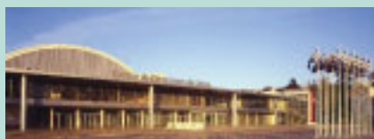
The Congress Centre of Lisbon: all facilities one can imagine
